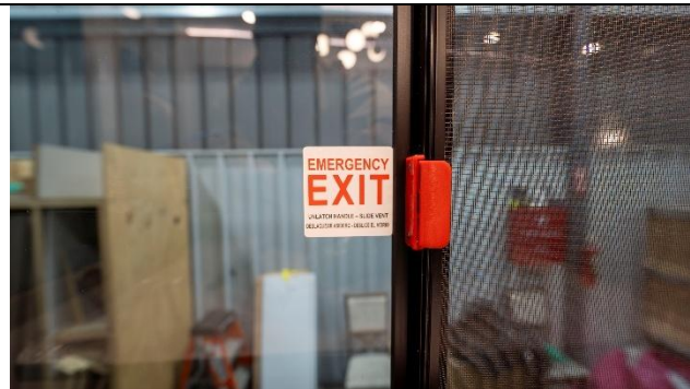
Figure 8. Pull style latch on an emergency exit.
