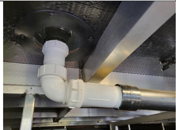
Figure 63. Waterless p-trap under a shower location.
