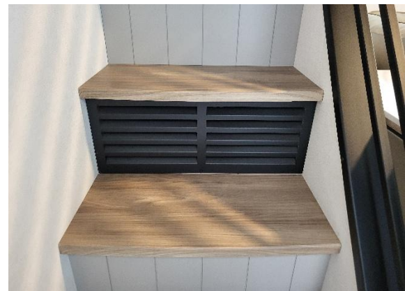
Figure 58. Louvered panel on rear stairs. Remove this panel using the 6 screws to access the sanitizing and winterizing valves and plumbing.
