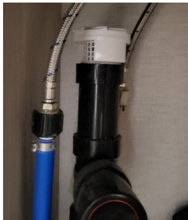
Figure 64. Air admittance valve.
