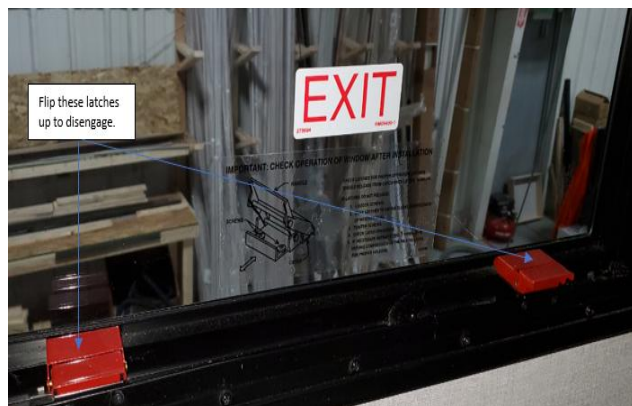
Figure 10. Flip style latch on an emergency exit.
