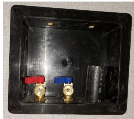
Figure 69. Washer connections and drain.
