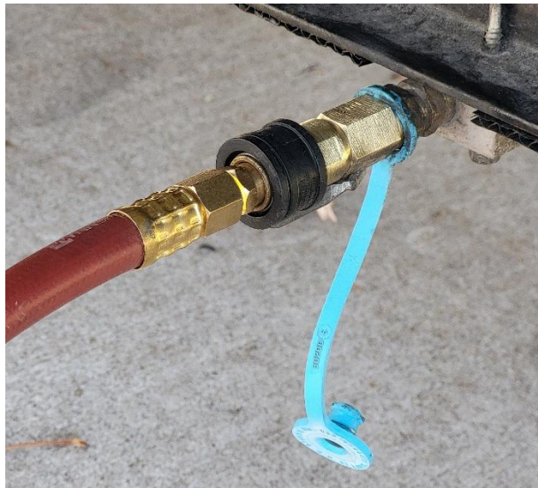
Figure 20. Connected appliance, with flow lever rotated forward to the "on" position.
